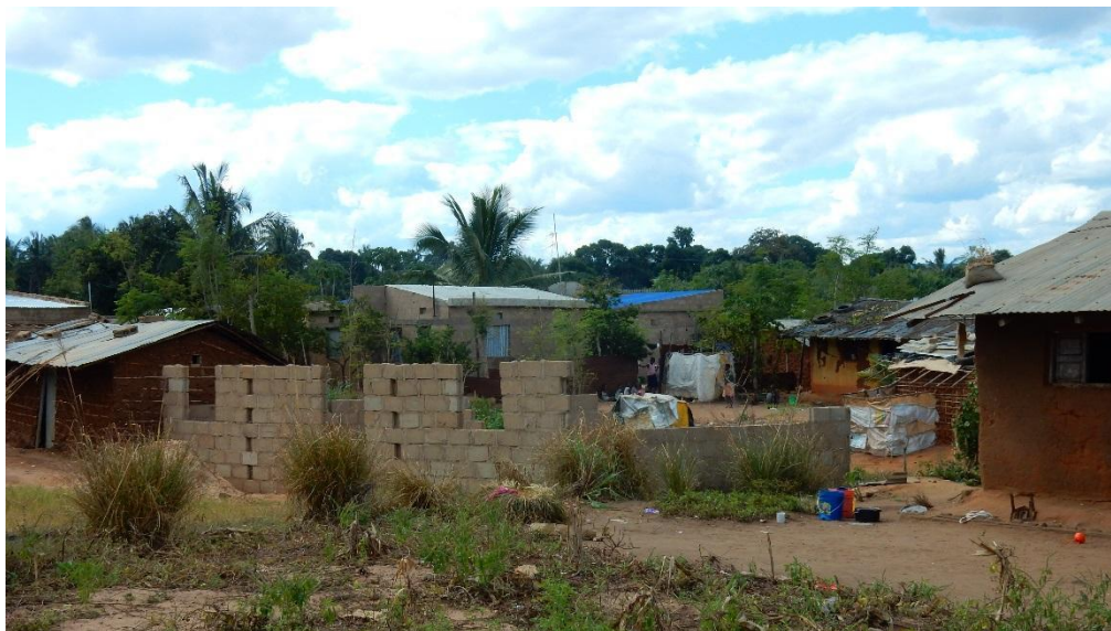
Figure 35: Unfinished construction - Nampula, 2016
